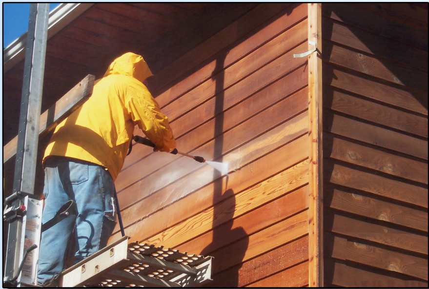
Lightly pressure wash to rinse off Clean & Brite
